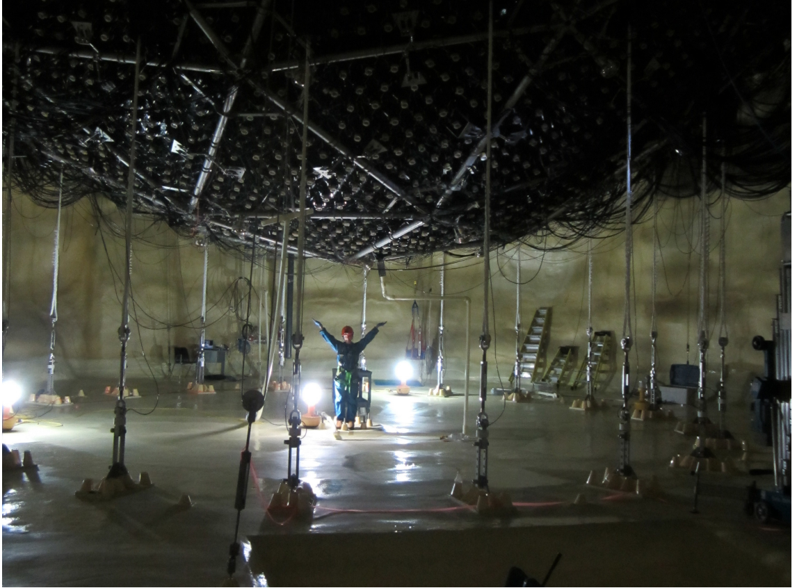
Figure 3.11: View from the base of the cavity, showing the rope net anchored to the cavity floor.
