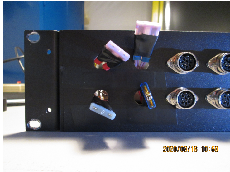
Figure 3.28: A picture of the TELLIE fuses after isolation work, March 2020.
